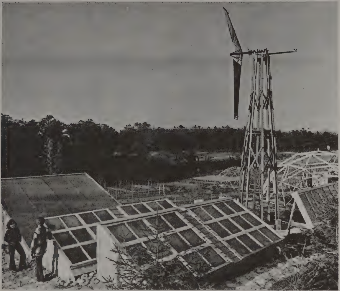
The Mini-Ark, a closed-loop stream. At right, the solar water heater. Foreground, the bio-purification unit and supplemental food sub-ecosystem. To the left, the polyculture fish pond and terrestrial plant greenhouse. The sailing windmill has a reciprocating rod leading downward to a wooden box pump (which outperforms and outlasts commercial plastic pumps). The windmill lifts the water in the "stream" to its highest point.
